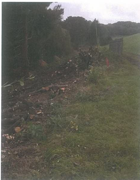
Photo: Tree clearance work at the site
