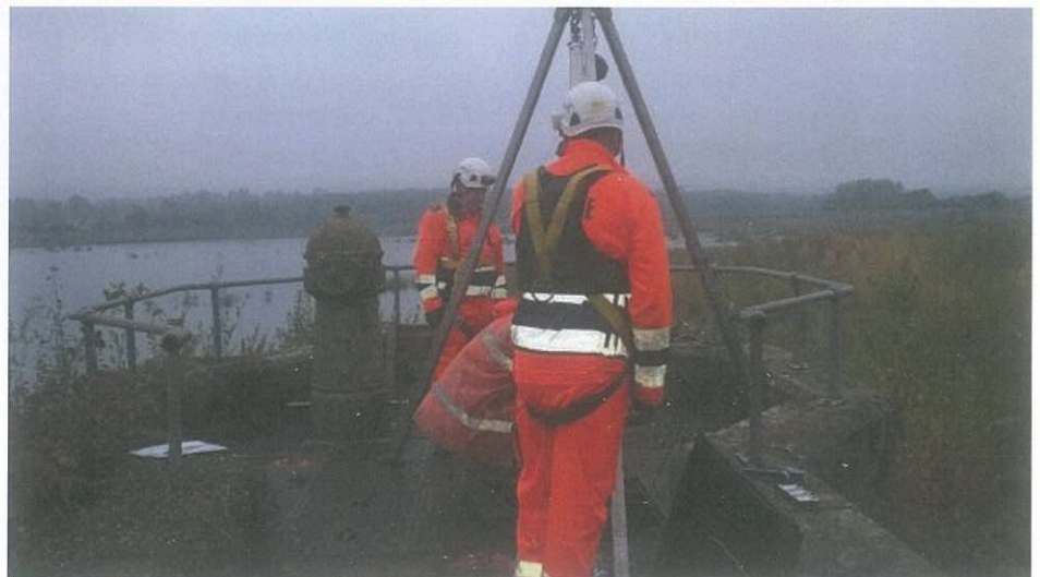
Photo: Specialist engineers working on one of the reservoir chambers
